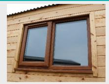
The doors and windows that we use are doubleglazed units and manufactured to the same high standards as those fitted into houses. Internally finished in white and externally finished in brown wood grain. Each window has an opening pane with lock and key to provide ventilation and the door has a security lock.
