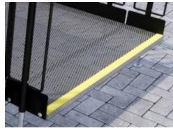
Contract bands are a safety feature to identify the nose of the ramp or step and any changes in level or gradient.
