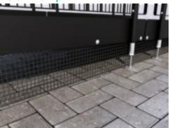
Mesh infill is designed to prevent unauthorised access and stop litter from blowing underneath the ramp.
