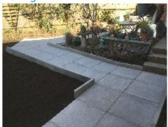
Paving can be used in conjunction with modular ramps or as a standalone ramp solution.
