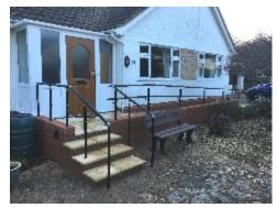
The same type of handrails as used on the modular components can be used as standalone rails. They can even be used to create a continuous rail across a transition from modular ramp to paved area for example.
