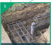
Straight sections and corners are designed in the reinforcing to fit the required foundation shape.
