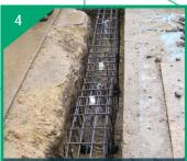
The reinforcing cages are manufactured off-site and simply lowered into position over the piles.
