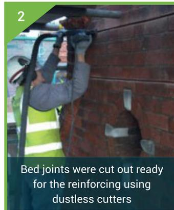
2 Bed joints were cut out ready for the reinforcing using dustless cutters
