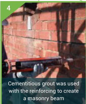
4 Cementitious grout was used with the reinforcing to create a masonry beam
