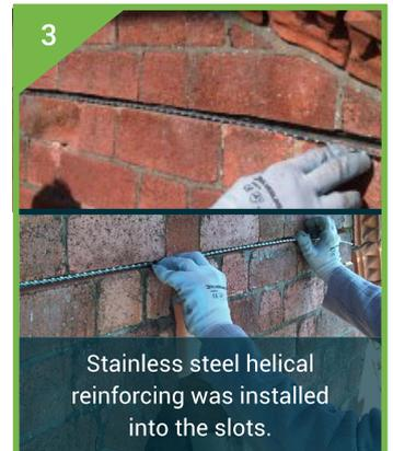
3 Stainless steel helical reinforcing was installed into the slots.
